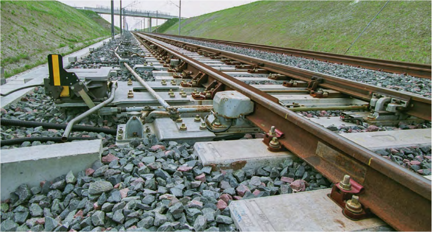
Figure 12 – A high speed turnout on the Paris to Strasbourg High Speed Line. Photo SNCF.
