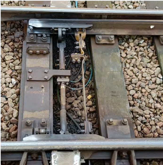
Figure 10 – Typical clamp lock installation. Photo Francis How.
